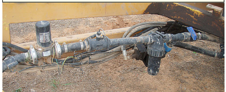
Below: From L-R Raven flow control valve, flow meter and 100mesh spray filter pump outlet, bypass tap.
