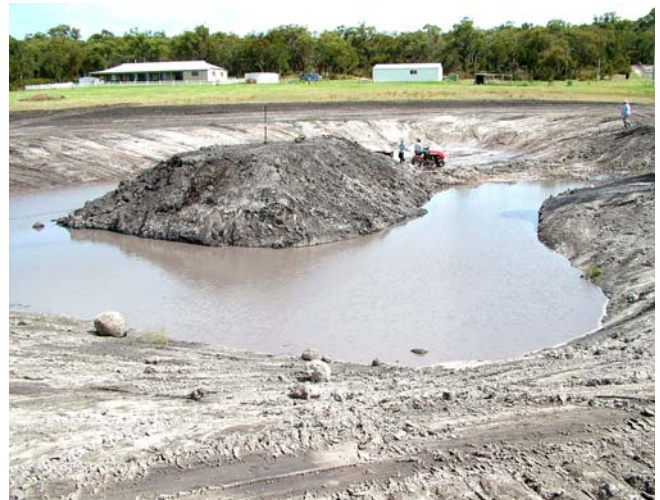
27 th Feb 2005. Our new dam in Paddock 1. It's filling up from seepage which is why we put the dam there.
